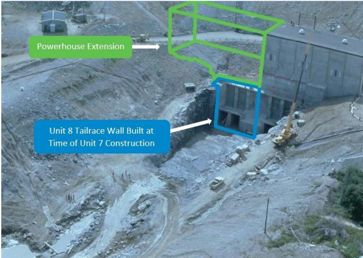
Figure 6: Original Powerhouse 2/Unit 7 Construction with Provision for Unit 8
